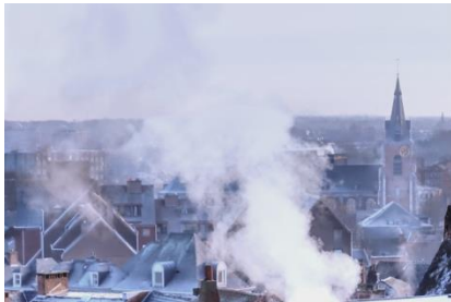
All excess heat to City of Joensuu's district heating network
